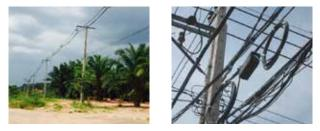
GTS; ALT's subsidiary, offers services including site survey, design and fiber optic cable installation (outside plant), either backbone network installation interconnecting regional exchange locations with thousands of kilo-meter distance, or within the regional network installation, to connect the exchanges within a region which is less distance. Scope of works regarding to this service are;
